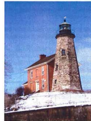
The Charlotte Lighthouse is a symbol for the surrounding neighborhood as well as a historic landmark. Photo: ZHA, Inc.
