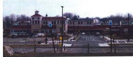
Figure 13. Ferry Terminal Building
