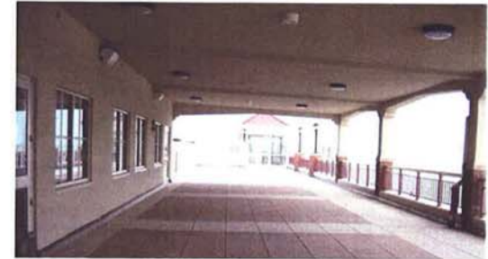
Figure 10. Terrace looking down river to lake
